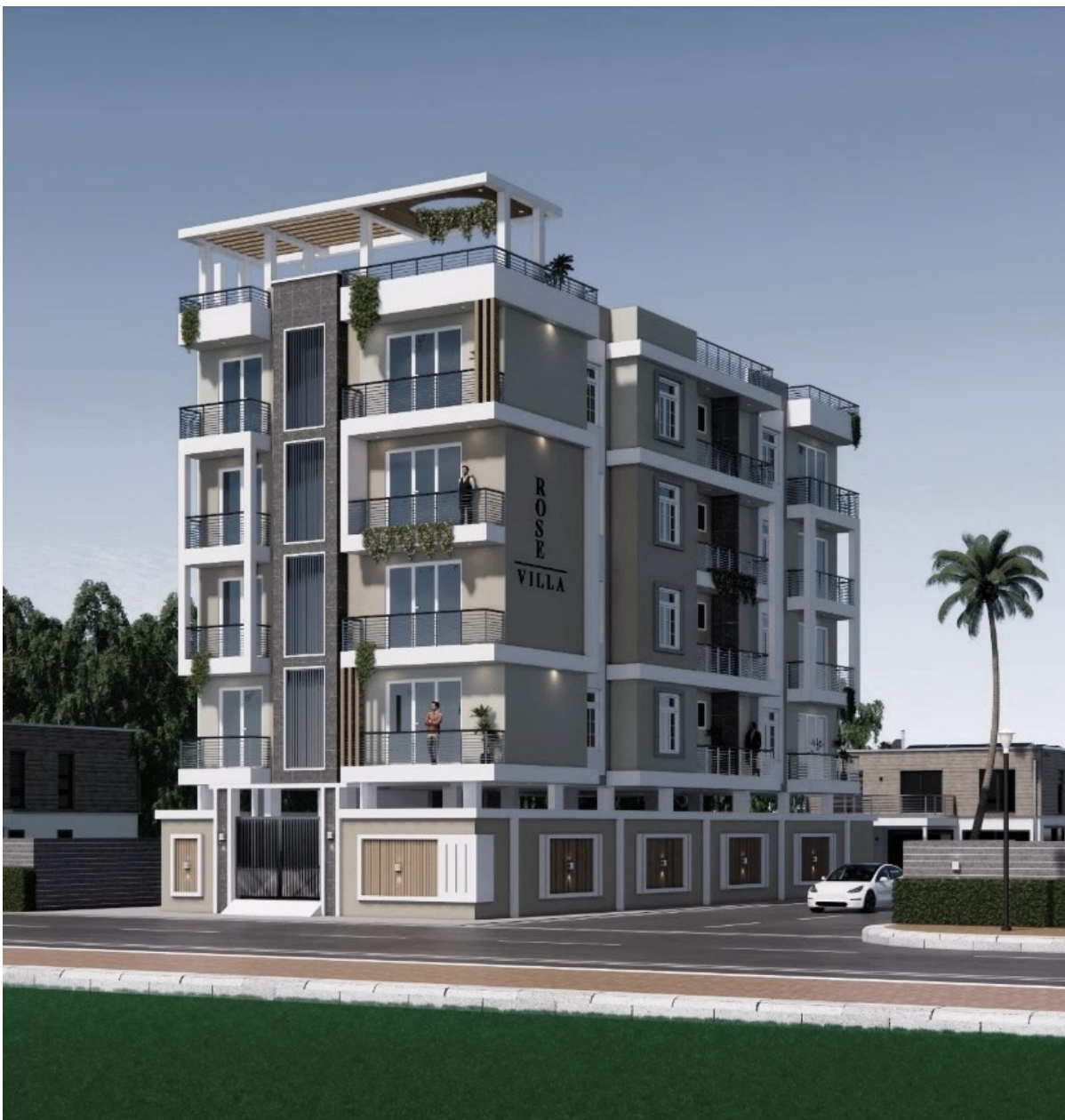
Figure 34- Case study building
