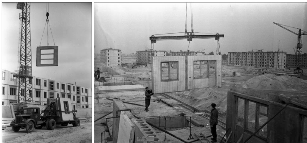
Figure 1 - Prefabricated panel construction in 1960, in Ukraine (Malaia, 2020)
