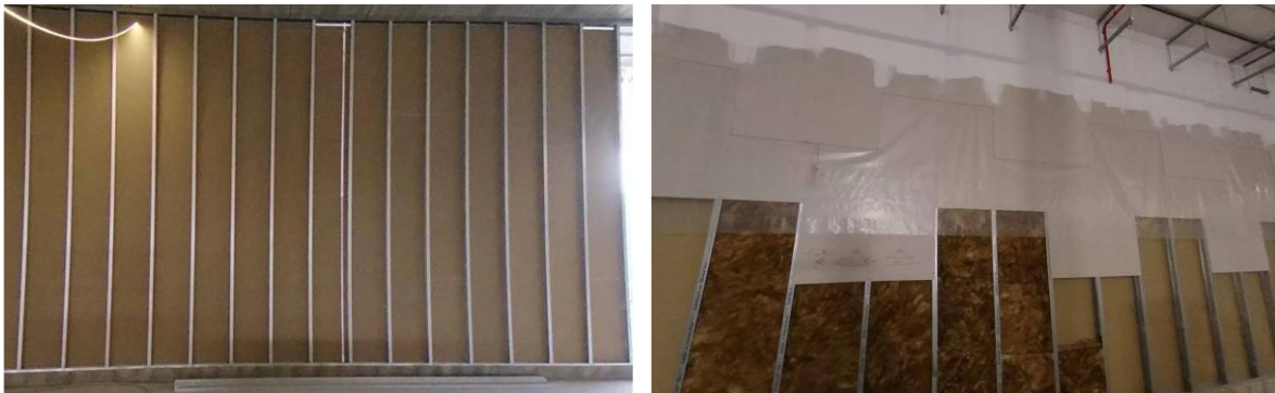
Figure 6 – Class C wall example photos
