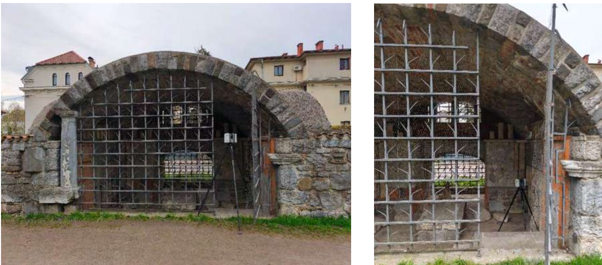
Figure 78 Capturing the positions that will allow the stitching of the inside and the outside point clouds.
