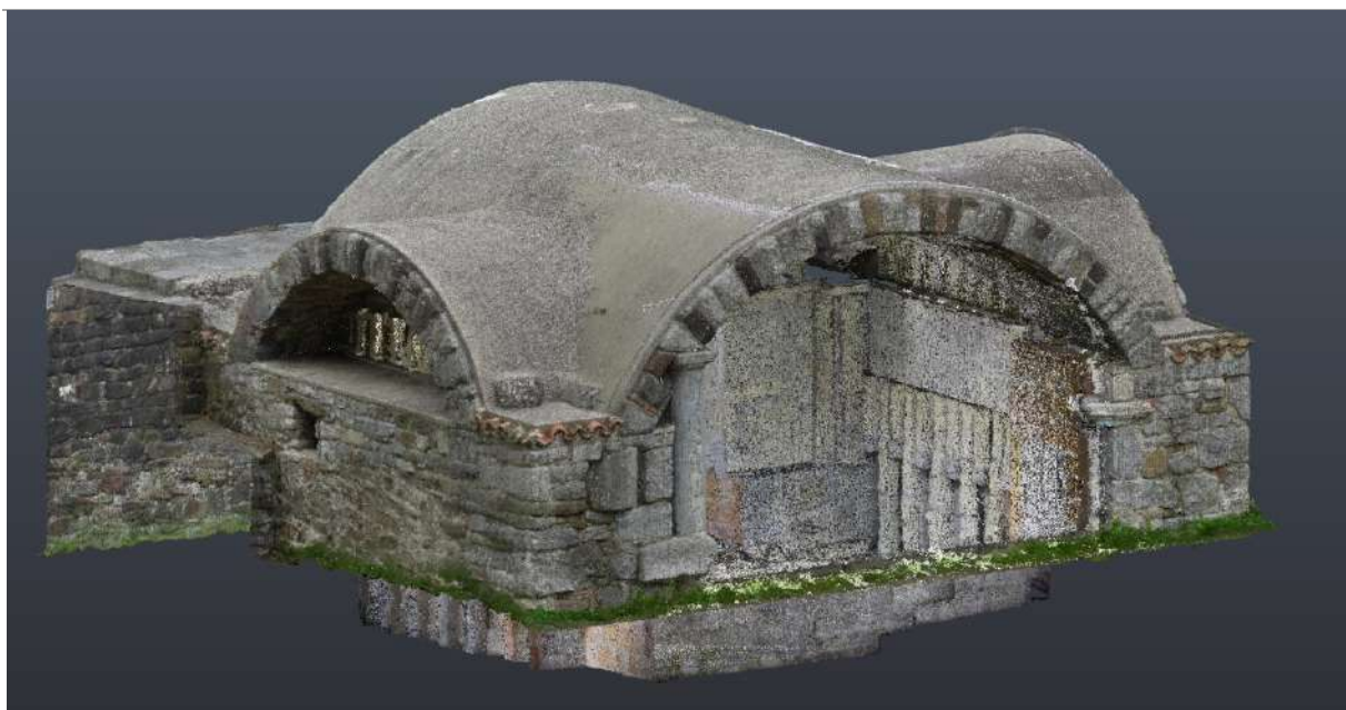
Figure 35 The Lapidarium LIDAR interior dataset after manual cleaning and stitching to the outside in the correct geographical position.
