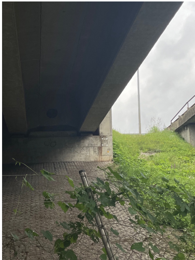
Figure 20: Wing – Viaduct B.
