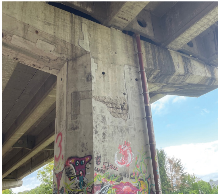
Figure 25: Retrofit on Pier 6 – Viaduct A.
