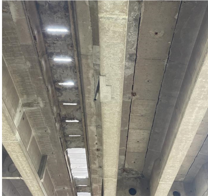
Figure 26: Retrofit on Girder group 4 – Viaduct A.
