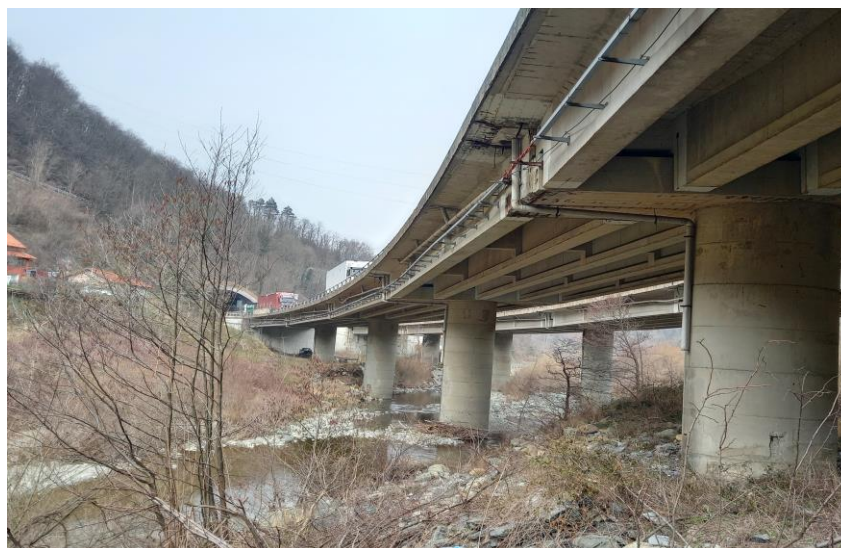
Figure 4.2 – San Pietro Bridge (Bottom)
